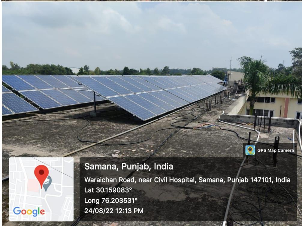
**35 KVA Roof Top Solar Power Plant installed in the College**
